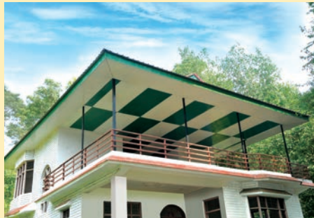
Terrace False Ceiling
