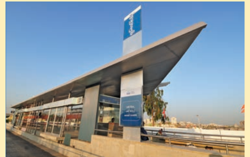
Bus Stop False Ceiling
